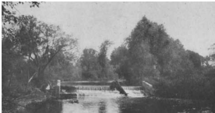
Old Mill Dam at Stuart's Flats on Whiteman's Creek, Burford
